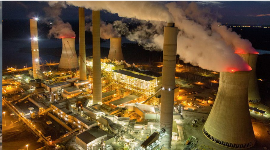
US coal power plant in Virginia
