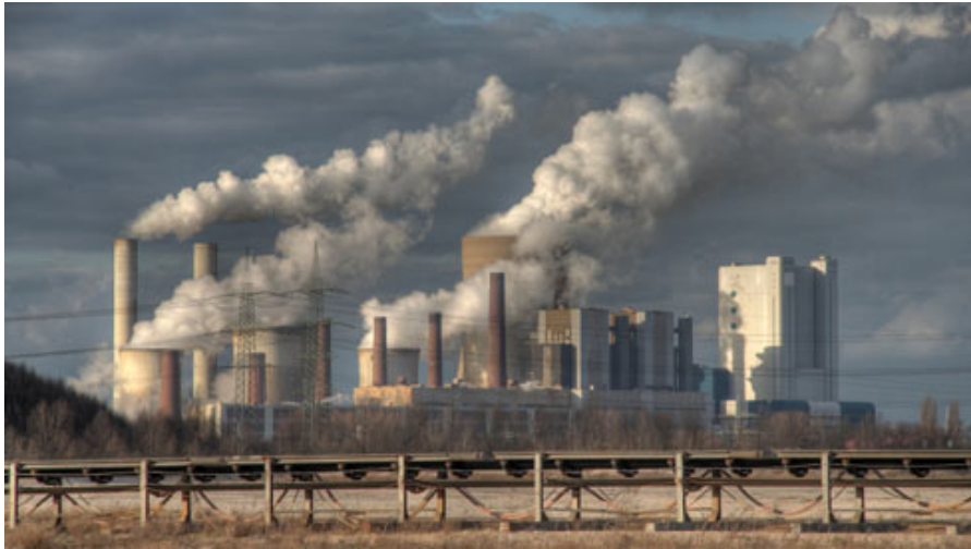
US coal power plant in Kentucky
